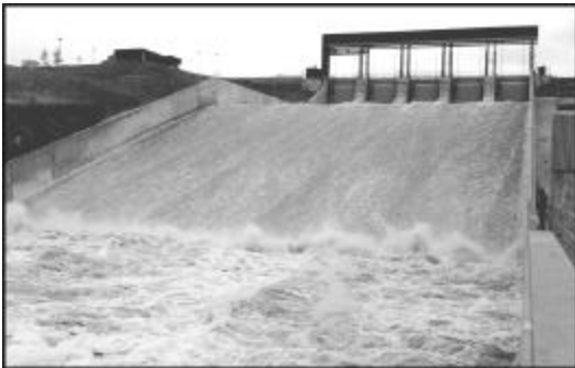
Dickson Dam Spillway
